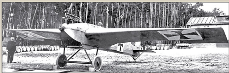
The original 120hp Daimler-Mercedes D.II powered steel skinned Junkers J 1 photographed on 12 December 1915.
