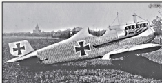
160hp Daimler-Mercedes D.III powered Junkers J 7 photographed on 12 October 1917 after it's rotating wing tips had been replaced by more conventional ailerons. Note the radiator mounted above the engine and style of exhaust manifold. Although not legible in this print, the wheel covers carry "Junkers & Co Dassau" markings.
